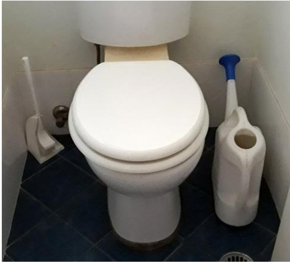
Collection vessel in place
