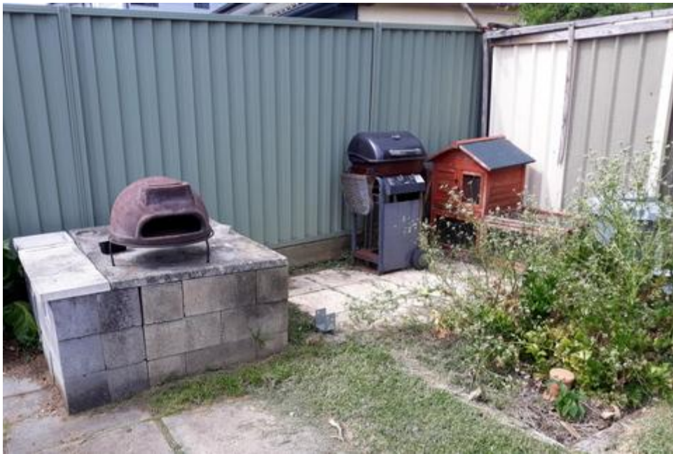
The area prior to cleaning and demolition
