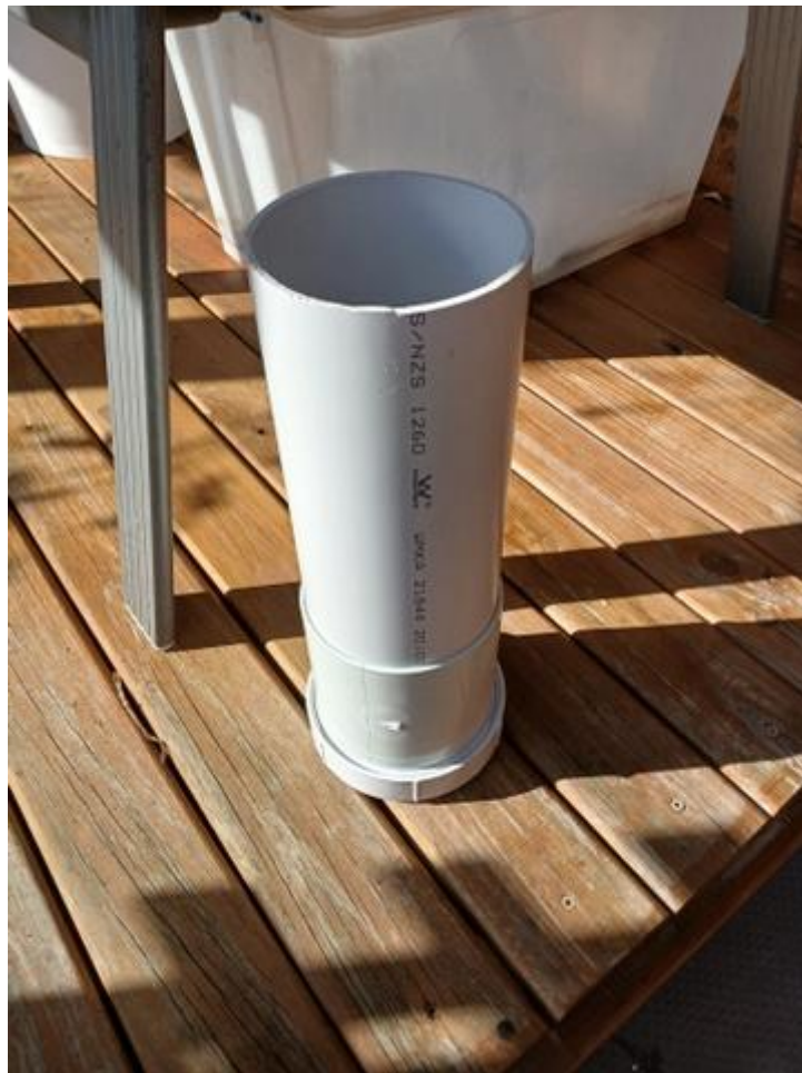
With the rest of the pipe inserted
