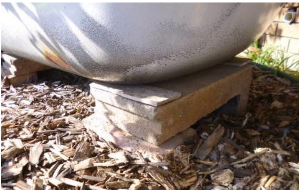
Supporting the first tub
