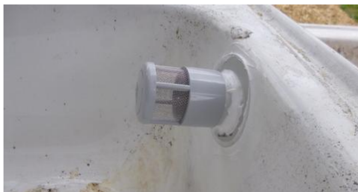
Attachment of the 50mm mozzie proof vent
