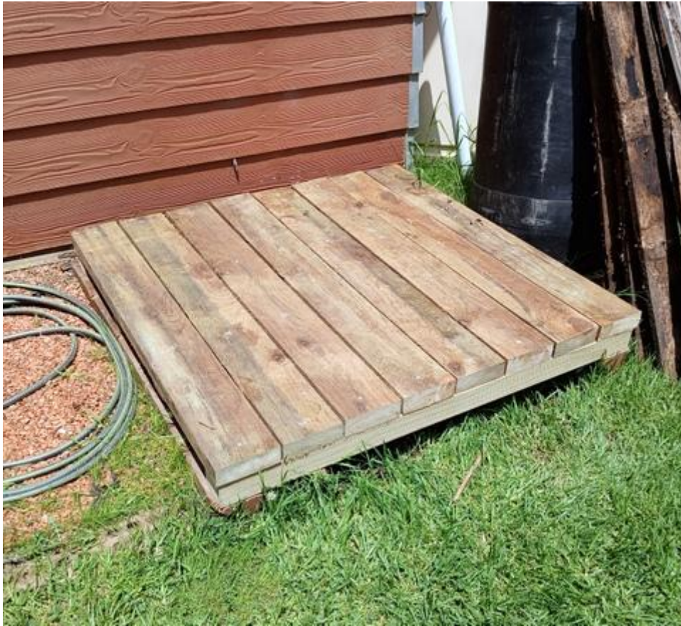
New timber base in place
