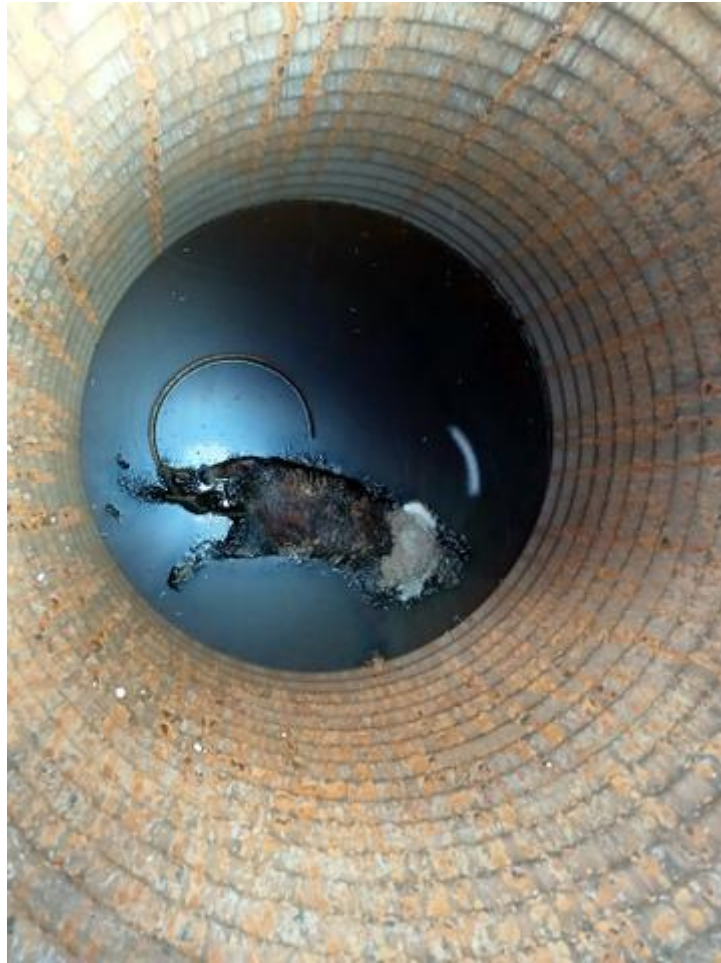
Tank c/w corpse (what appears to be along round tail is the rim of the galvanised disk sitting on the bottom of the tank)
