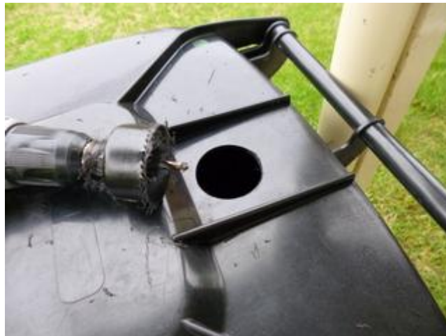
The hole in the top for the rainwater inlet
