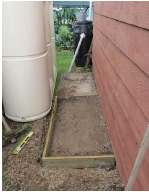
Tank delivered and sitting next to the under construction pad
