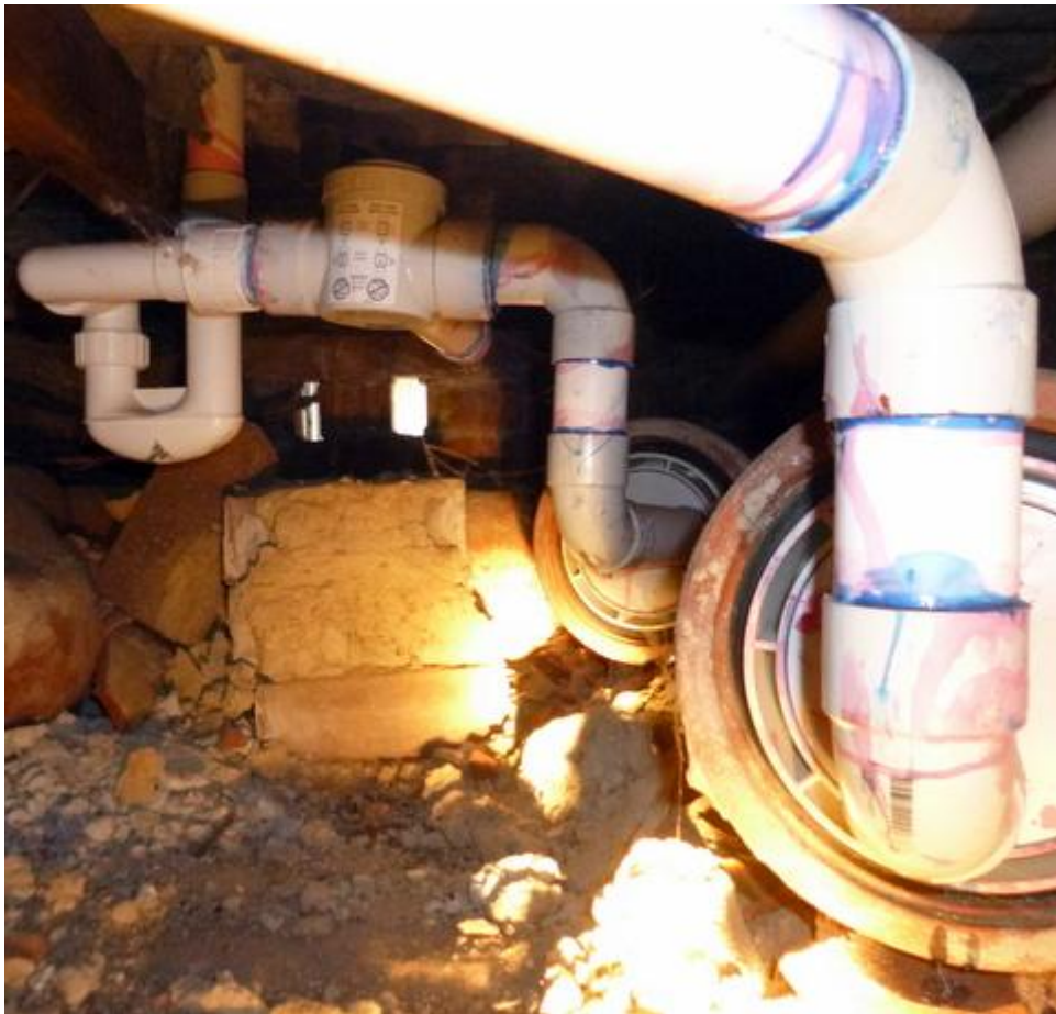
The original set up, with the drain from the spabath coming down, through the valve and over to the sewer
