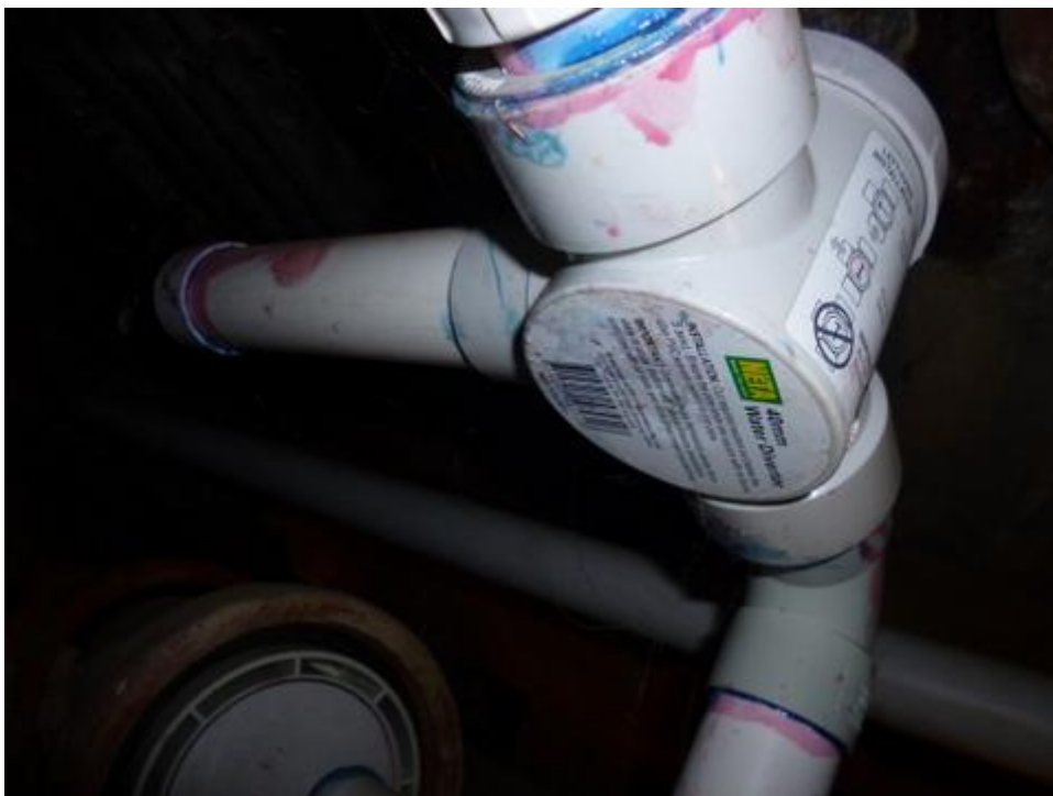
The original discharge pipe, blocked by a cap
