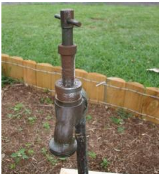
Fix those leaky taps!
