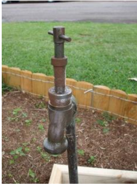
Tap reseater installed ready for use
