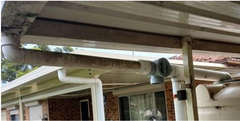
The original downward orientation of the valve outlet
