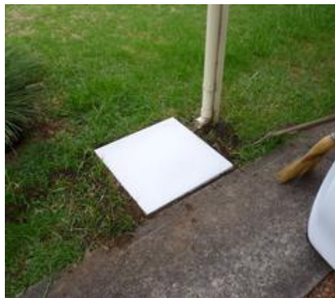
The concrete base in place
