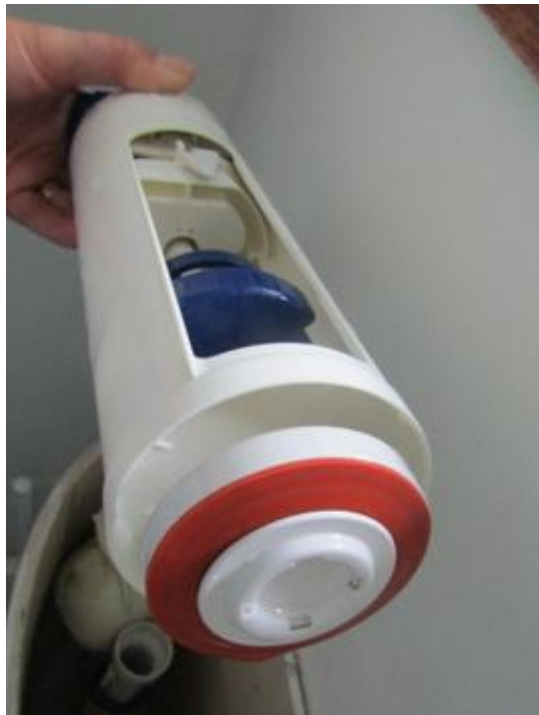
The orange flush valve washer at the base of the dual flush mechanism
