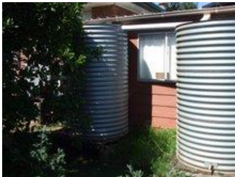
The original galvanised 2500 litre tanks
