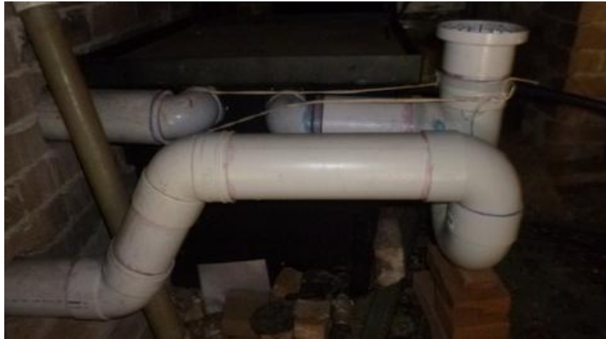
Pipes from the laundry and bathroom into the pit
