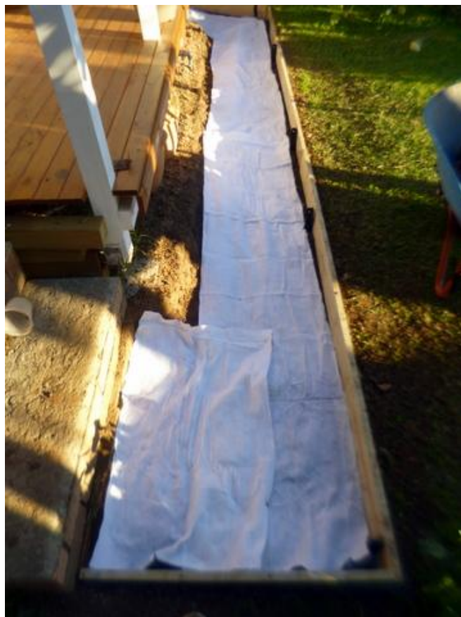
Dug out, with timber edging installed
