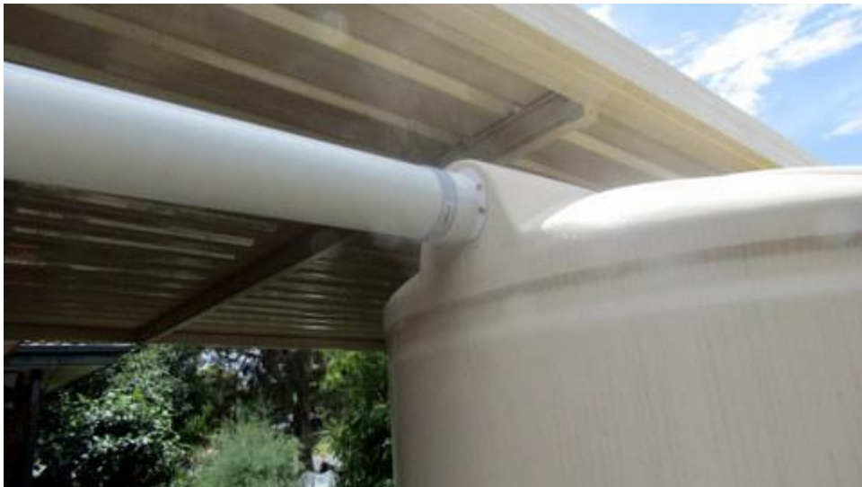
Drain from older tank fitted and plumbed in
