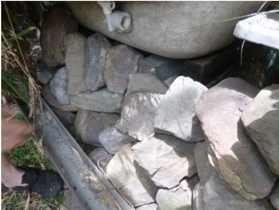
Support structure for spa
