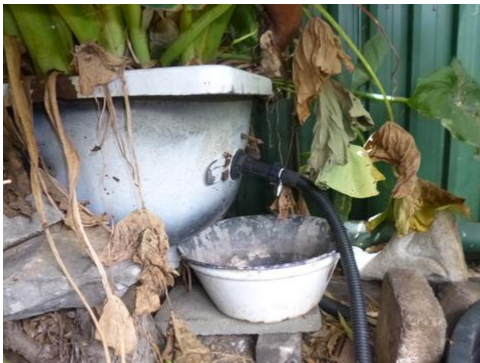
Water discharge from second bathtub onto soil via hose
