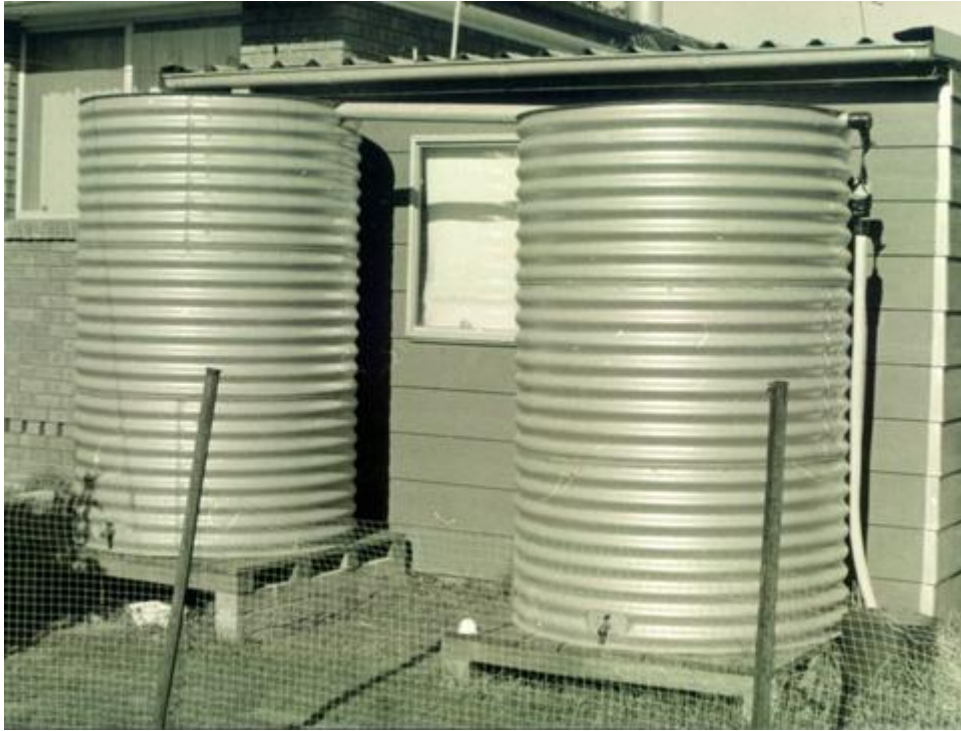
The original tank setup on the back of the garage
