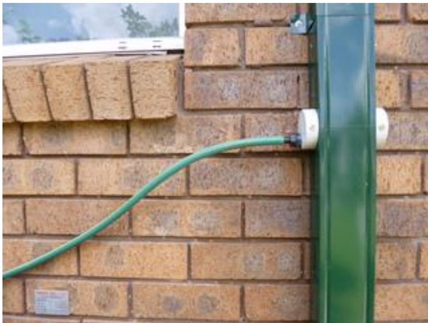
Hose in place
