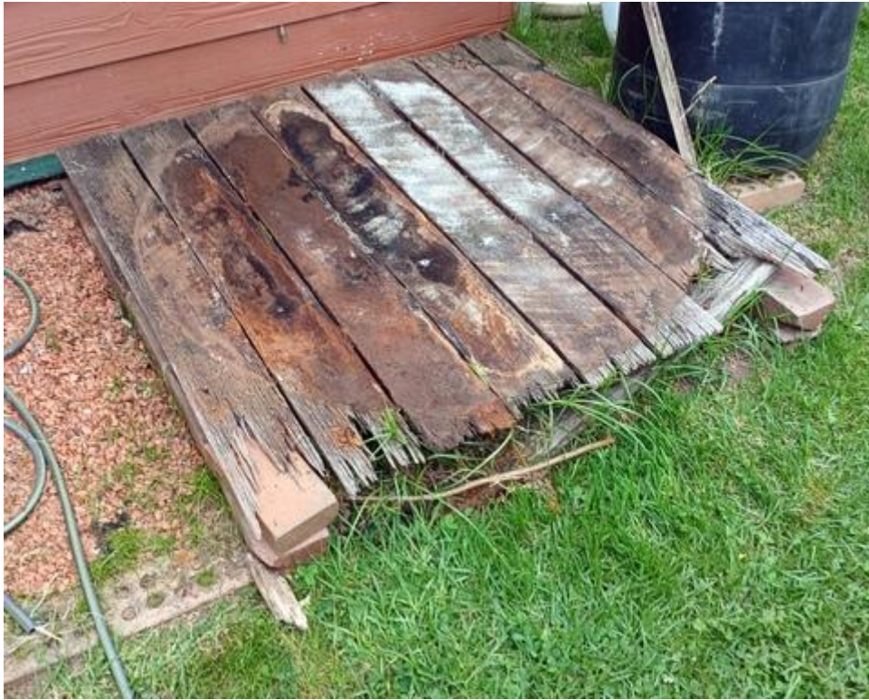
The original timber base. Not too bad, but not good enough to support a new tank!
