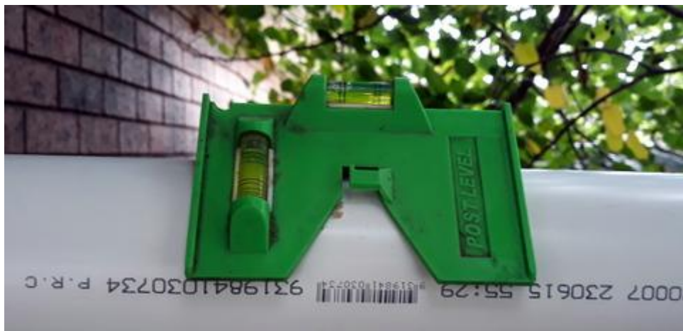
Making sure the drain has a slight down angle towards the tank
