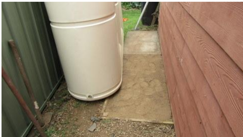
Bed prepared, moving tank over onto it
