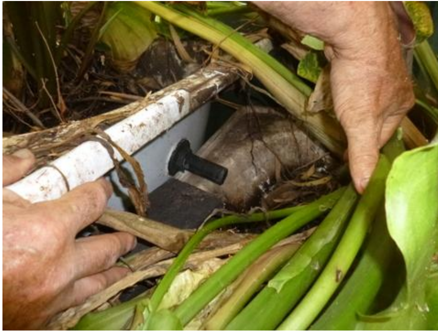
Drain from first bathtub into second bathtub
