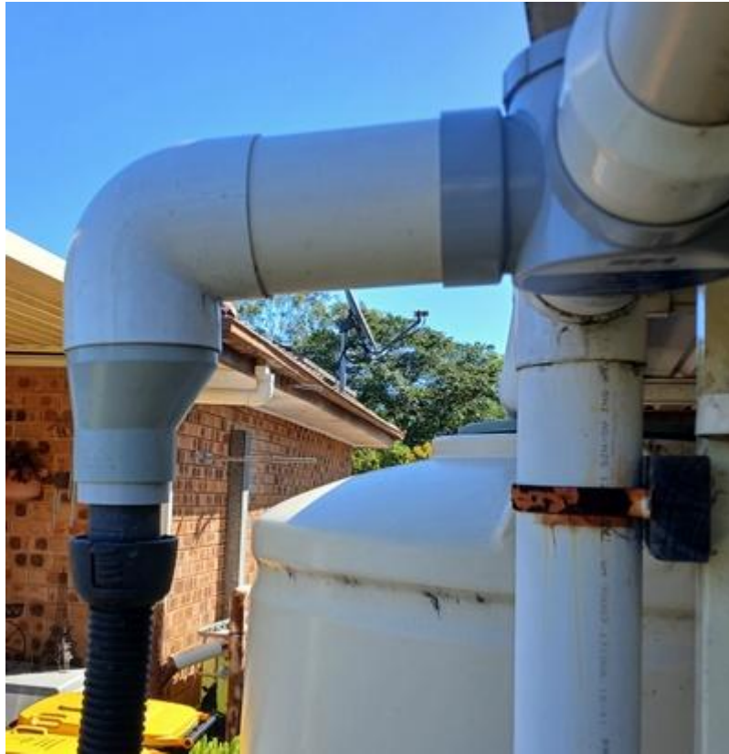
Final set up
