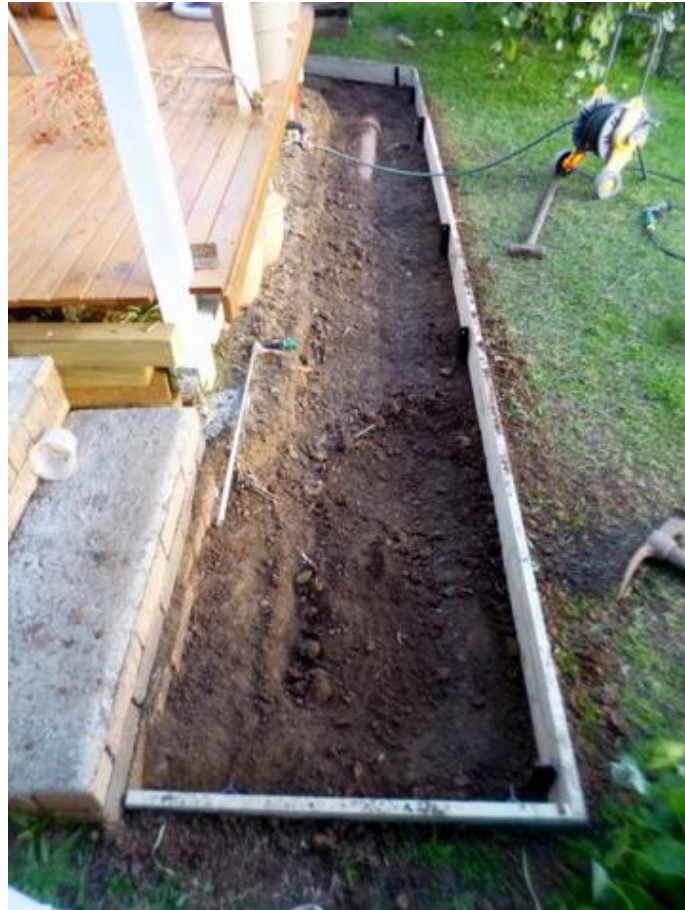
Dug out, with timber edging installed
