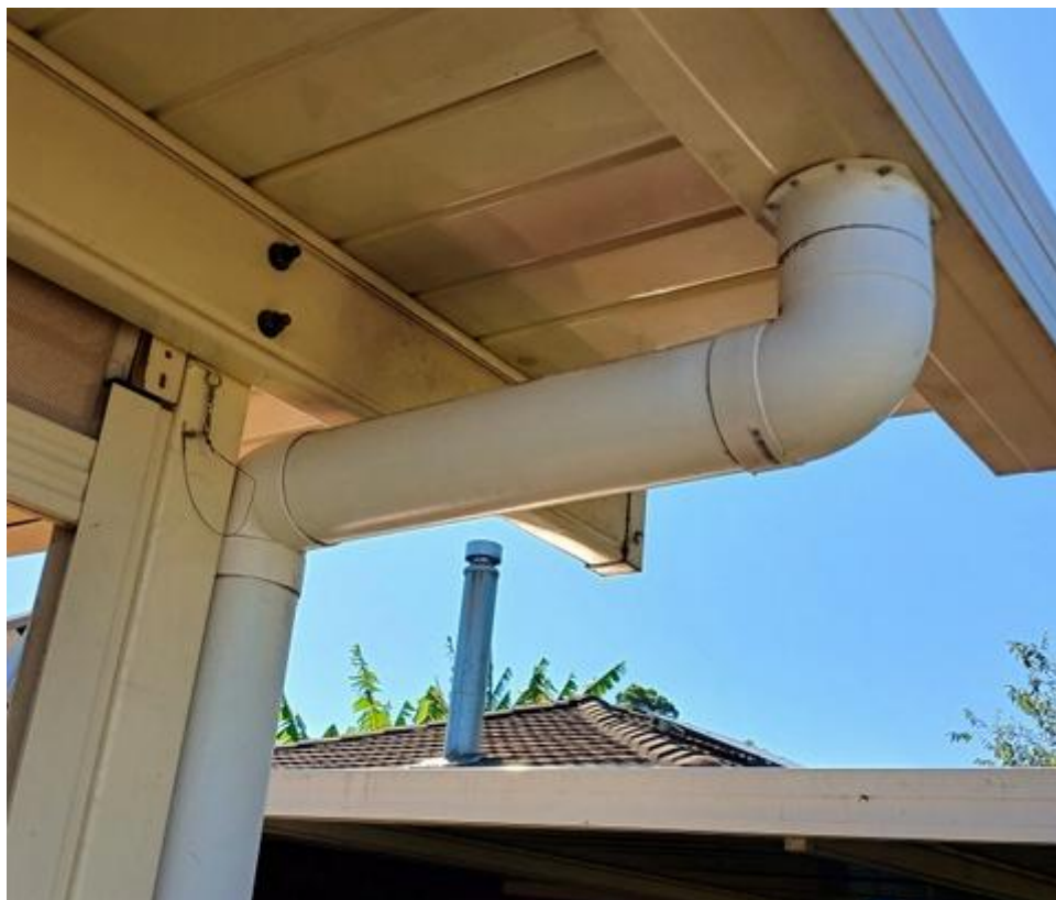
This section would be ideal for a first flush diverter
