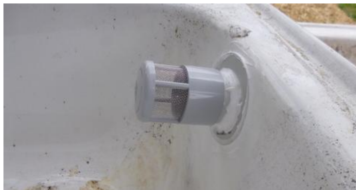
Attachment of the 50mm mozzie proof vent
