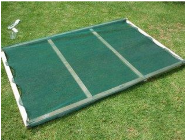
Frame bolted together and shade cloth attached
