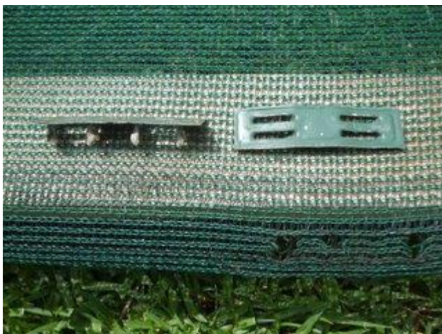
Detail showing gang nails used to attach shade cloth
