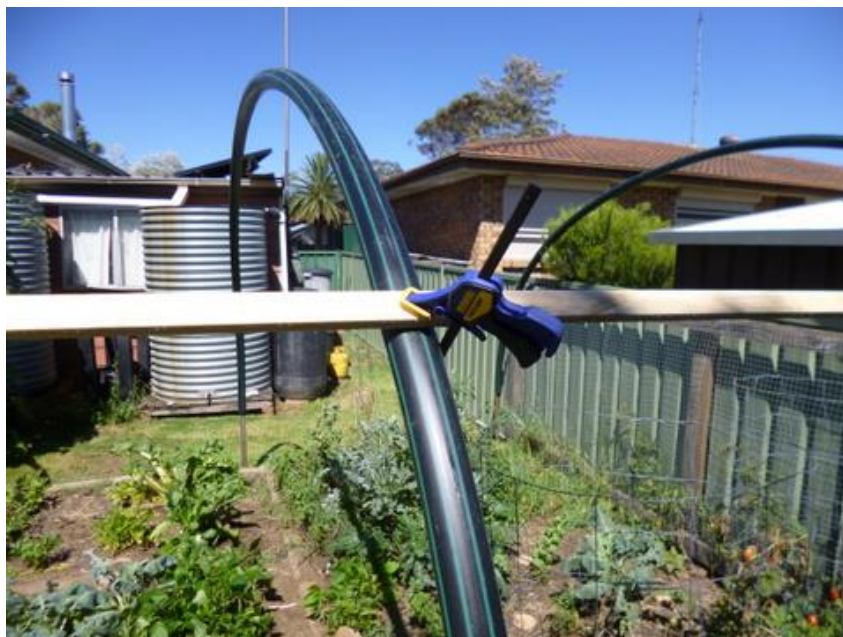
Holding the battens in place prior to fixing
