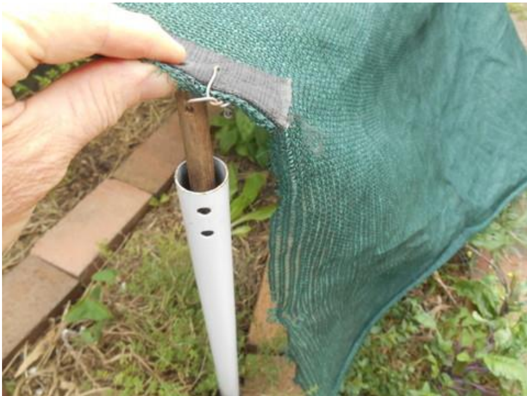
The dowel inserted into the support tube
