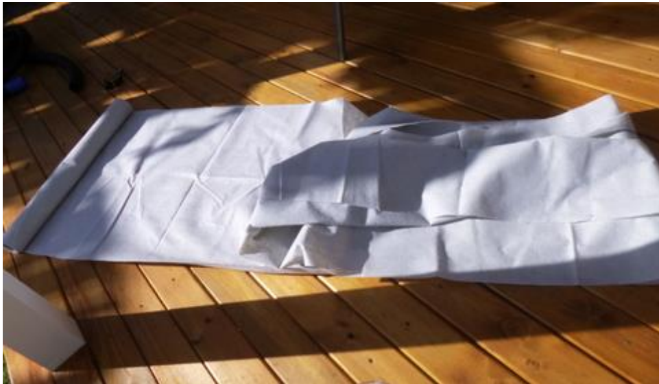
Drain Matting rolled out
