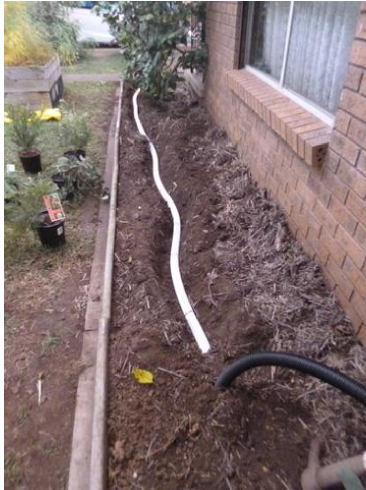
Buried pipe irrigation installed
