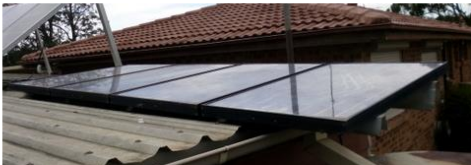
The bank of 4 Solarex panels for the fridge battery bank
