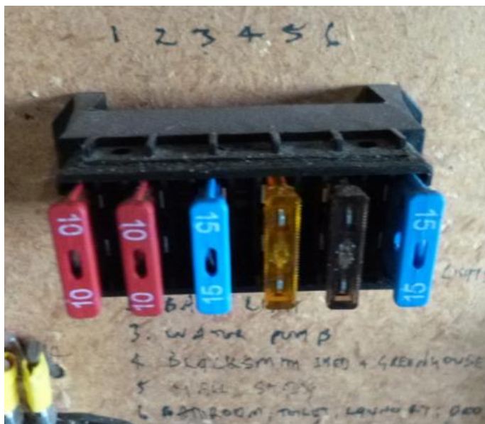
Fuse block and fuses
