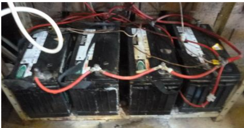
12 volt Superstart MF86B 130 amp hour marine maintenance free batteries
